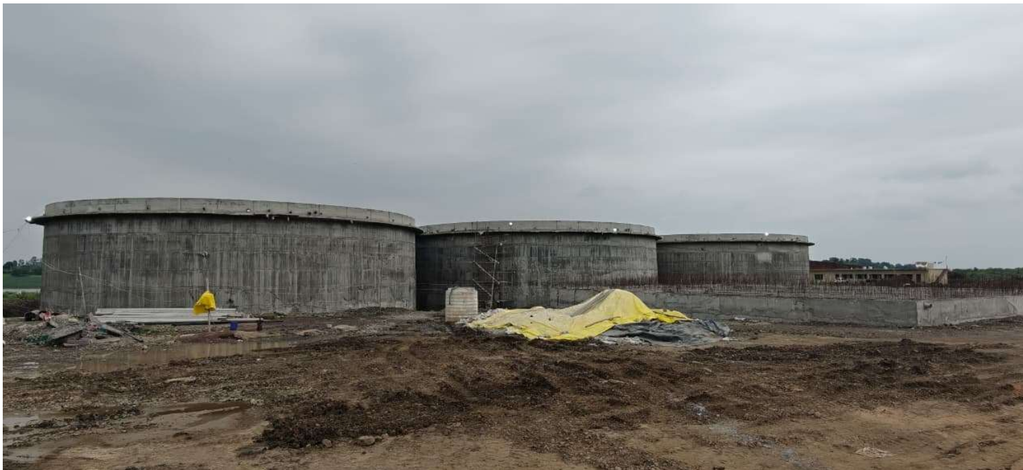
CBG Organics' plant under construction in Guna.
